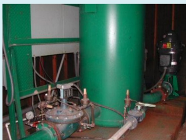
Conventional Pumping Station
